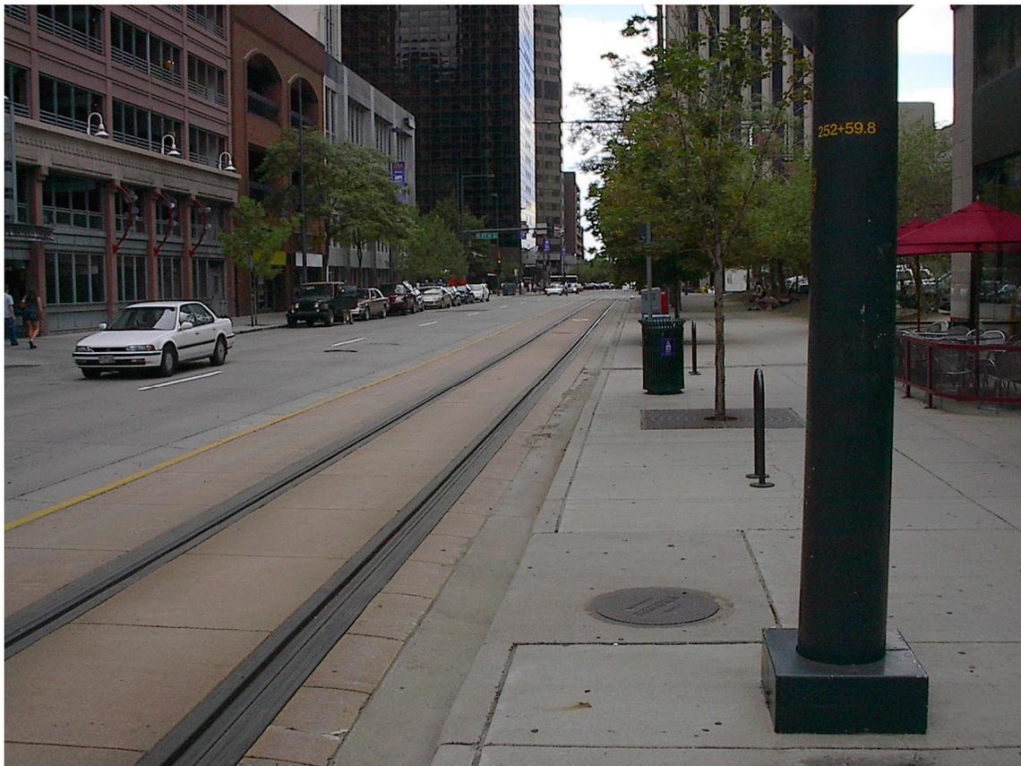
The above photo shows a typical downtown in-street LRT operation in Denver. The LRT trains are running counter flow to the direction of traffic on a one way street. Note the combined lighting/catenary poles, and physical differentiation between the LRT right of way and the adjacent roadway and sidewalk.
