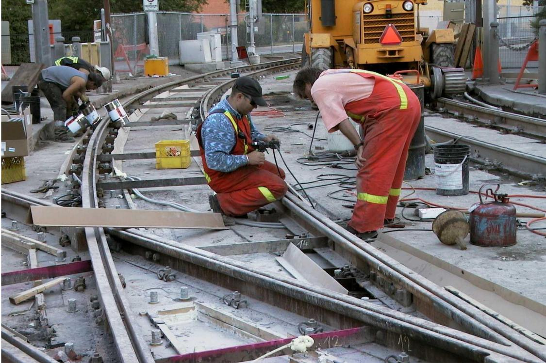
**Figure 7 - Calgary Transit LRT Staff Replacing Trackwork**
